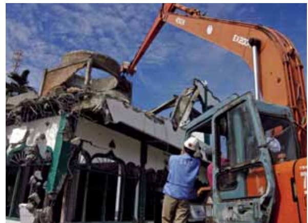
▼ Safe demolition of damaged buildings in Padang city. (UNDP Indonesia)
